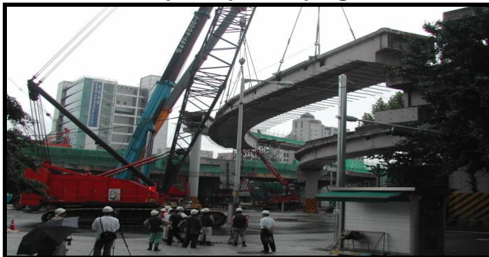
Cheonggyecheon restoration BOX-type GIRDER dismantle
