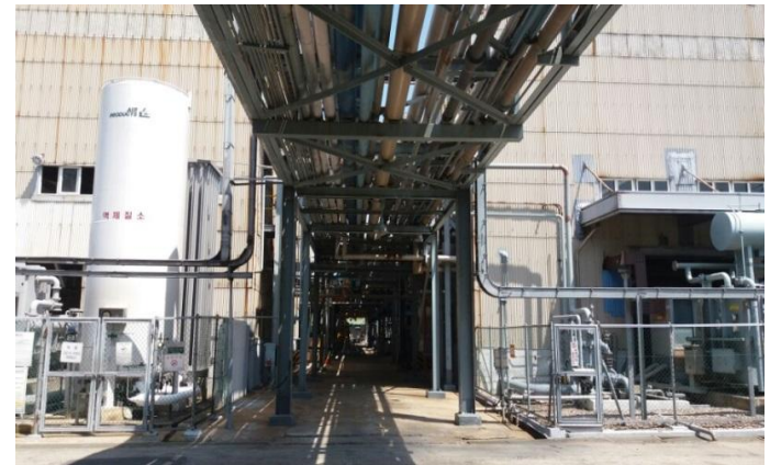
Ulsan Dongoh Chemical-Dismantle
