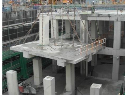
Dismantling offshore structure
