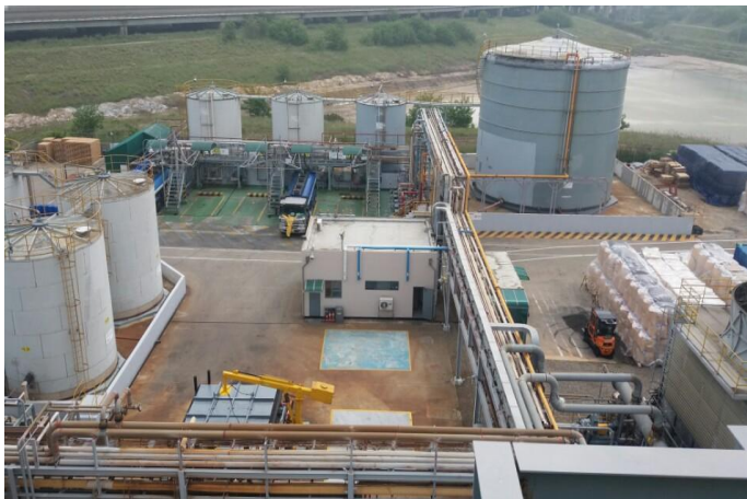
Ulsan Dongoh Chemical-Dismantle
