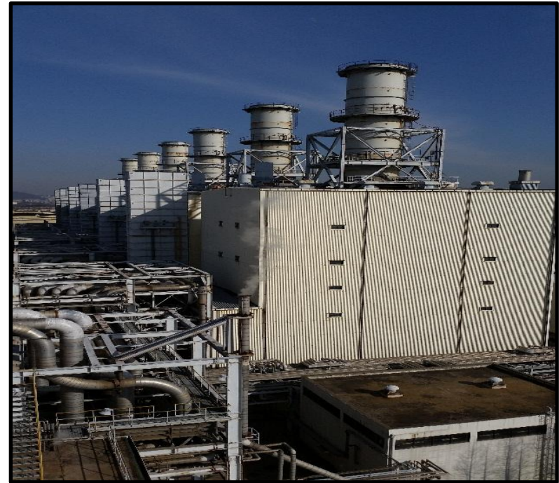
Posco Energy Incheon LNG Power Plant No.1,2 Dismantle
