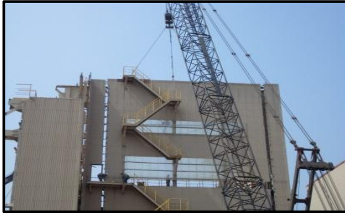
Posco Pohang Plant Test-CC Line-Dismantle
