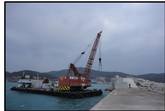
Chuja-do New Port Breakwater
