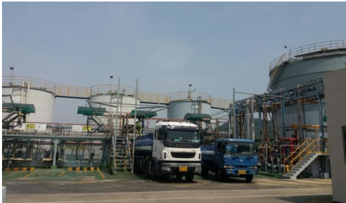
Ulsan Dongoh Chemical-Dismantle
