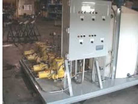
LCP Power off Confirmation and cable From To check
