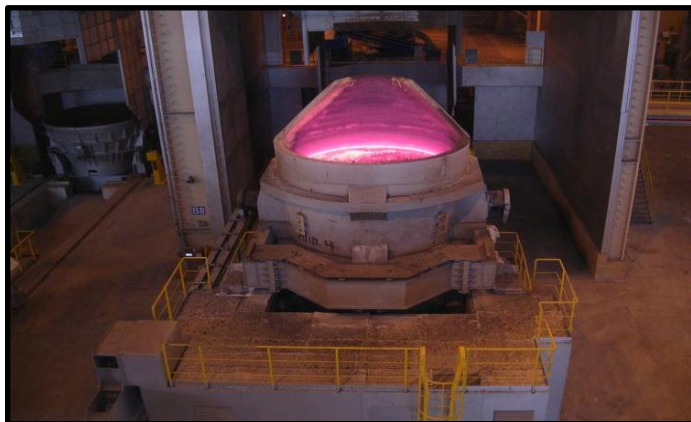
Posco Pohang Plant Test-CC Line-Dismantle
