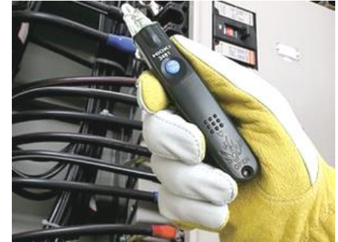
Check whether the equipment is energized by using non-contact type detector after wearing insulation protection
