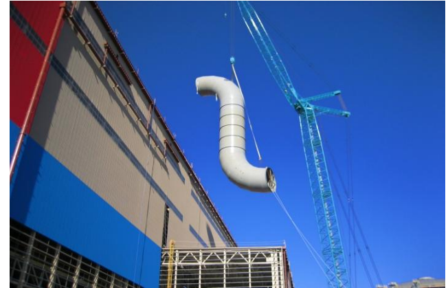
Posco Pohang Plant Test-CC Line Dismantle
