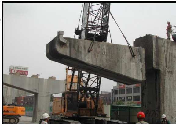
Cheonggyecheon restoration construction (Zone 3)
