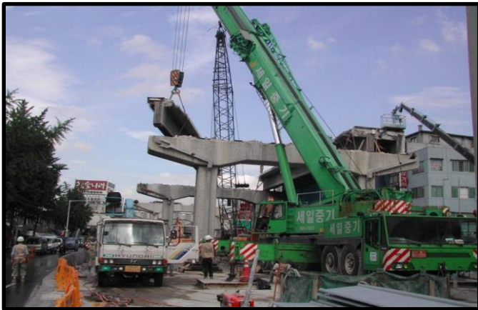
Cheonggyecheon restoration construction (Zone 1)
